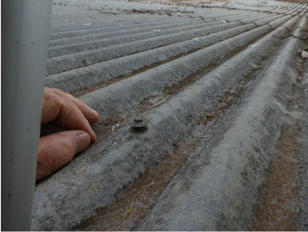
FIGURE 16; ROOF NAILS NEED ADJUSTING.
