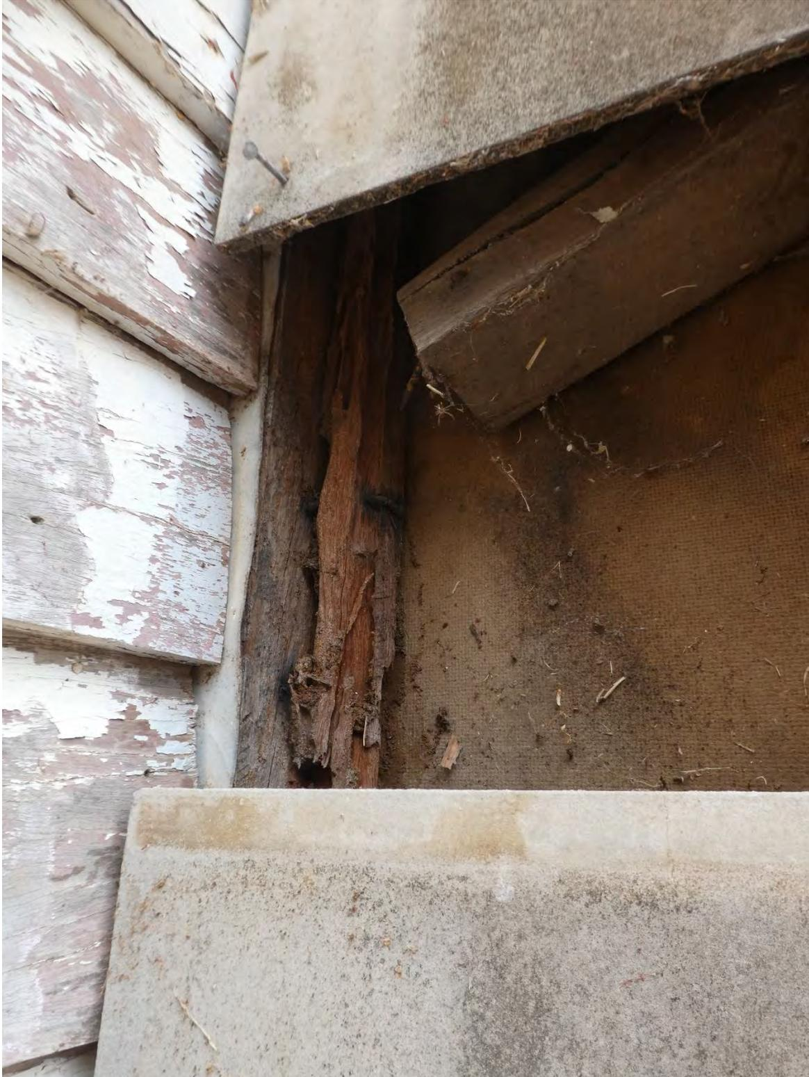
FIGURE 19; TERMITE DAMAGE.
