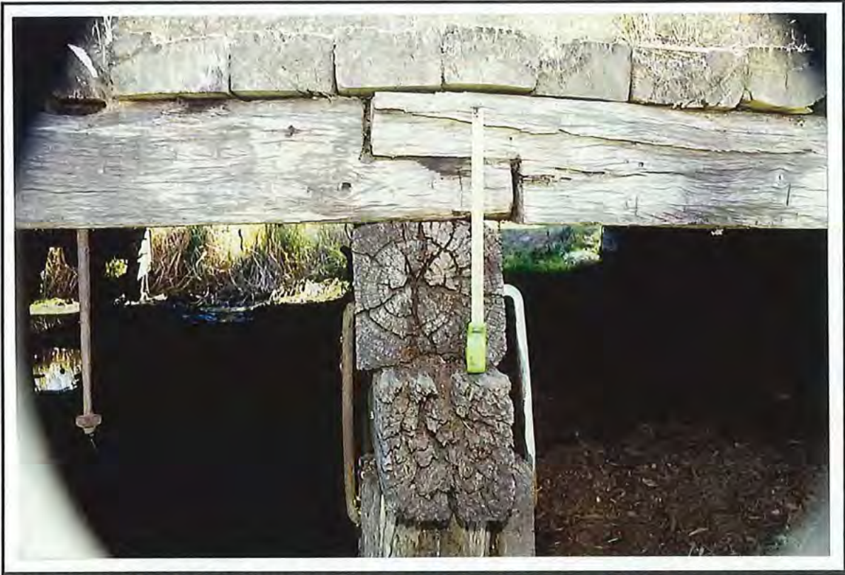
PIER 2 RIGHT HAND SIDE END CONDITION – NB OVER LAPPING STRINGERS
