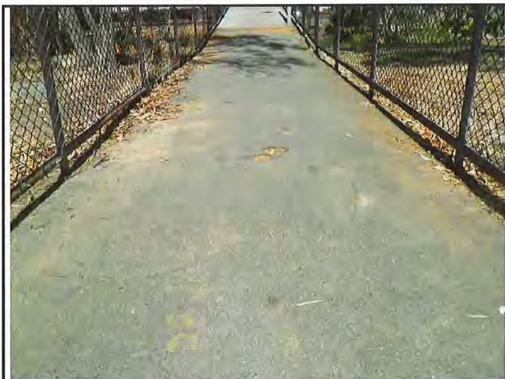
Photo No. 44: Surfacing A2 cracked
