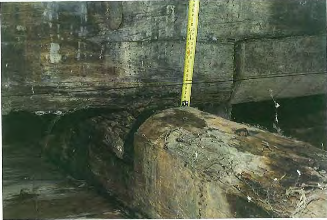
PIER 1 PILE 4 AT CORRECT HEIGHT
