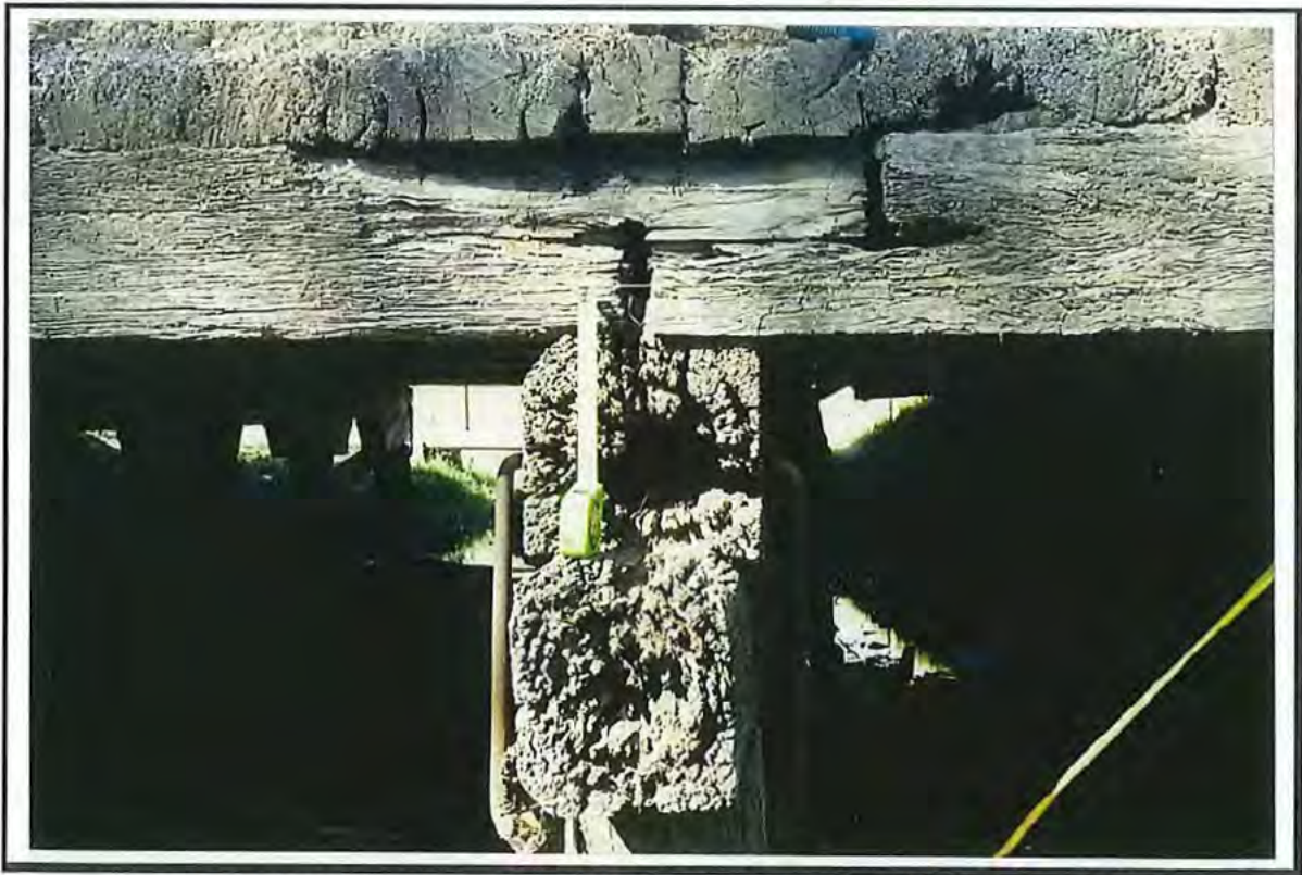
PIER 1 LEFT HAND SIDE SHOWING SUBSIDENCE 60-70MM FULL CAP CONDITION & CORBEL 1 LEFT HAND SIDE END CONDITION
