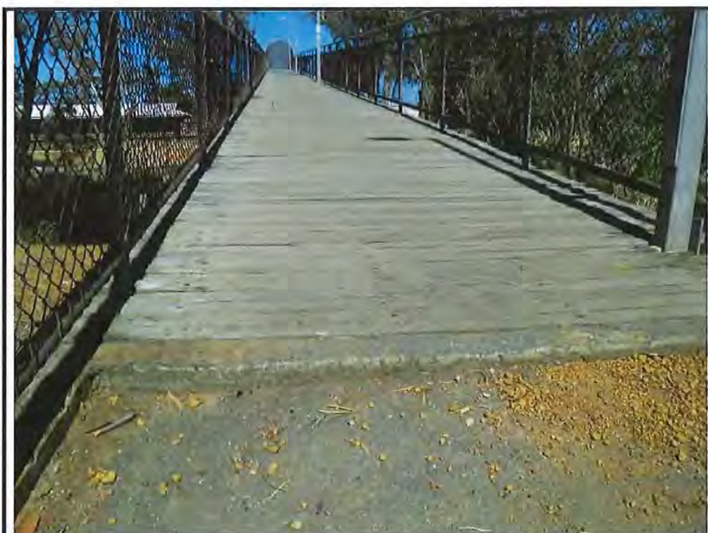
Photo No. 46: Minor trip hazard A2 end
