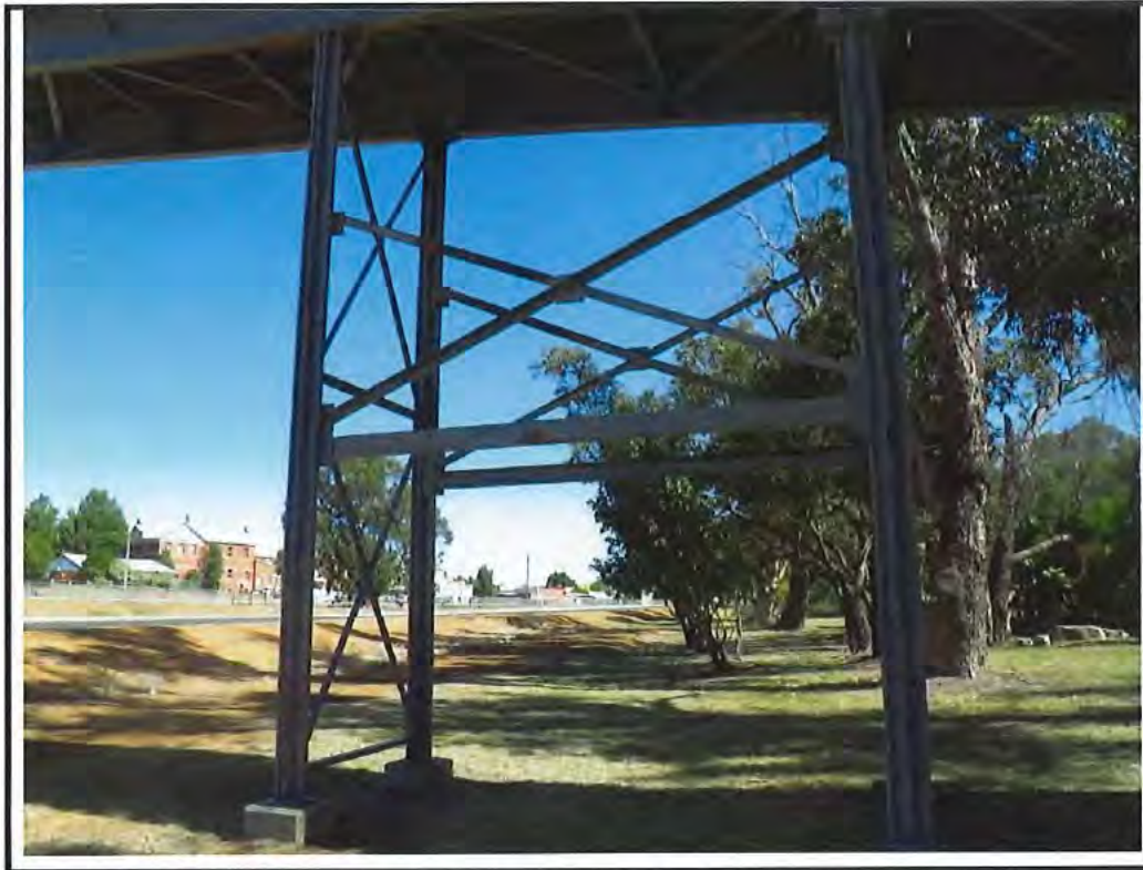
Photo No. 13: Bracing to Pier 5 and 6
