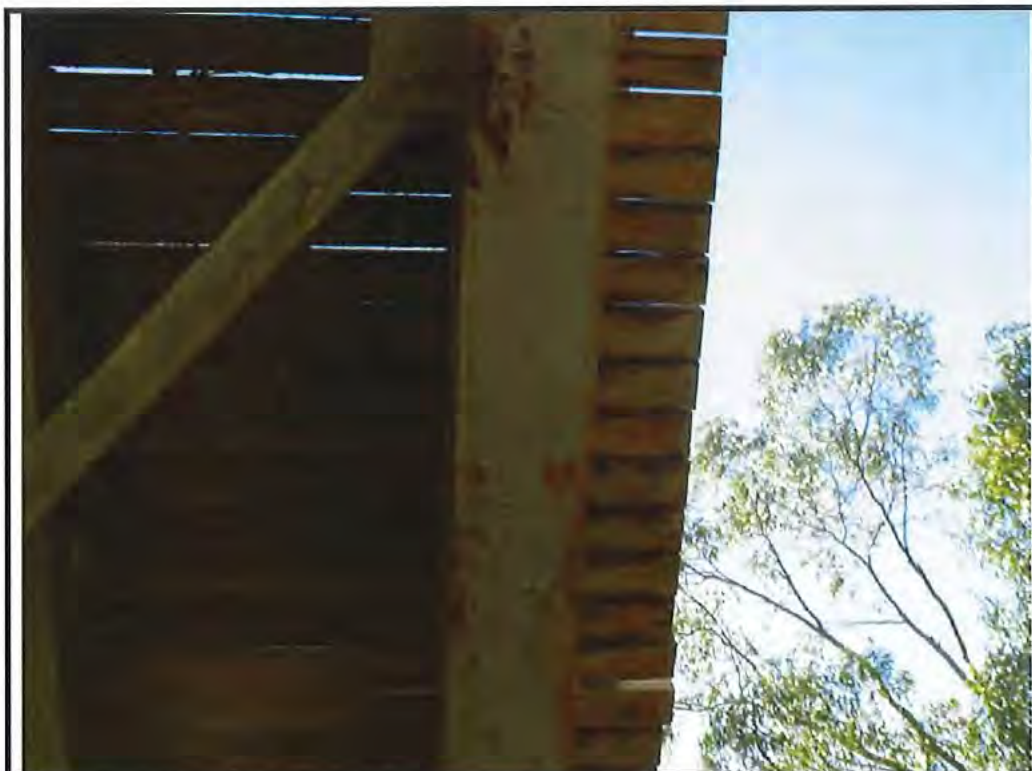
Photo No. 38: Minor surface corrosion to beams - typical
