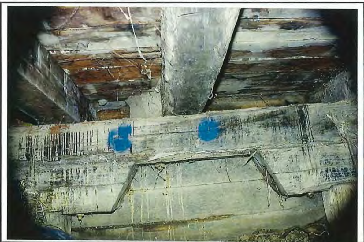
ABUTMENT 2 FULL CAP CONDITION BELOW STRINGERS 7, 8 & 9
