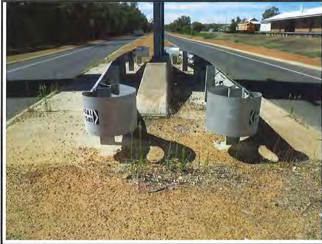
Photo No. 29: Inadequate pier protection – Pier 3
