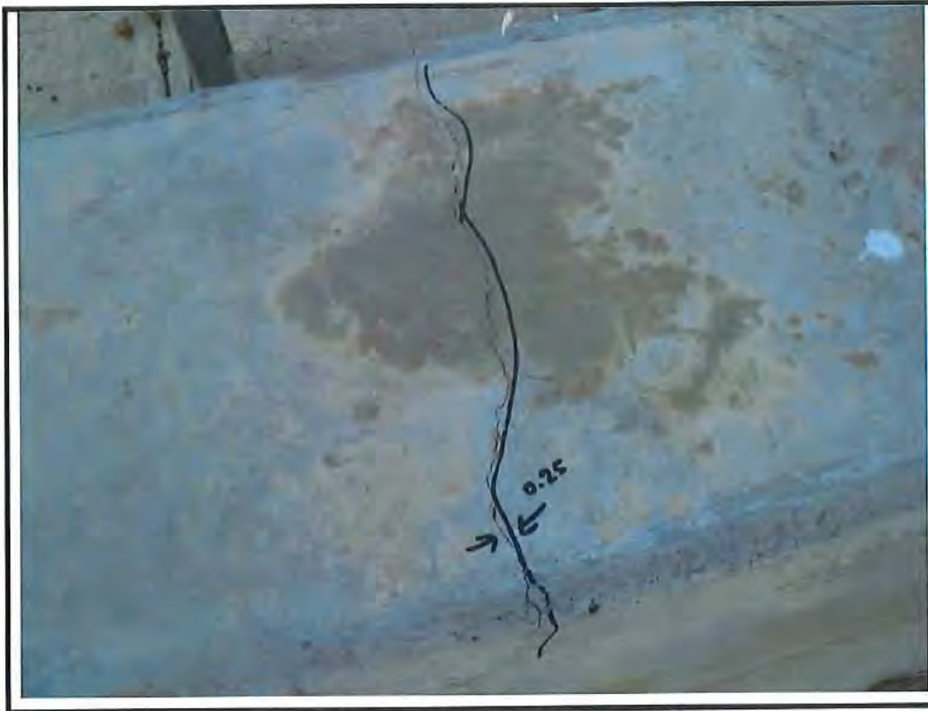
Photo No. 31: cracking to concrete surfacing Pier 3
