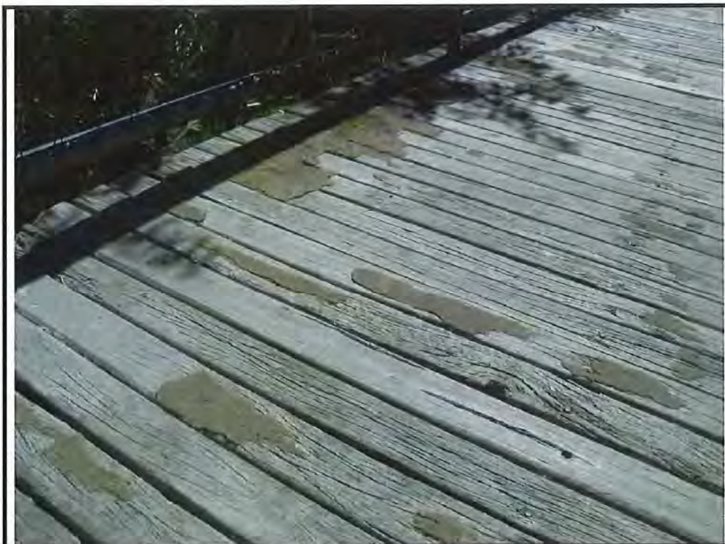
Photo No. 50: Anti-slip surfacing come of the ramp section of deck
