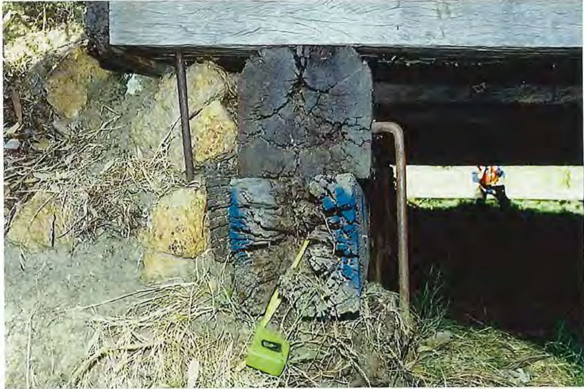
ABUTMENT 2 LEFT HAND SIDE FULL CAP & CORBEL 1 CONDITION
