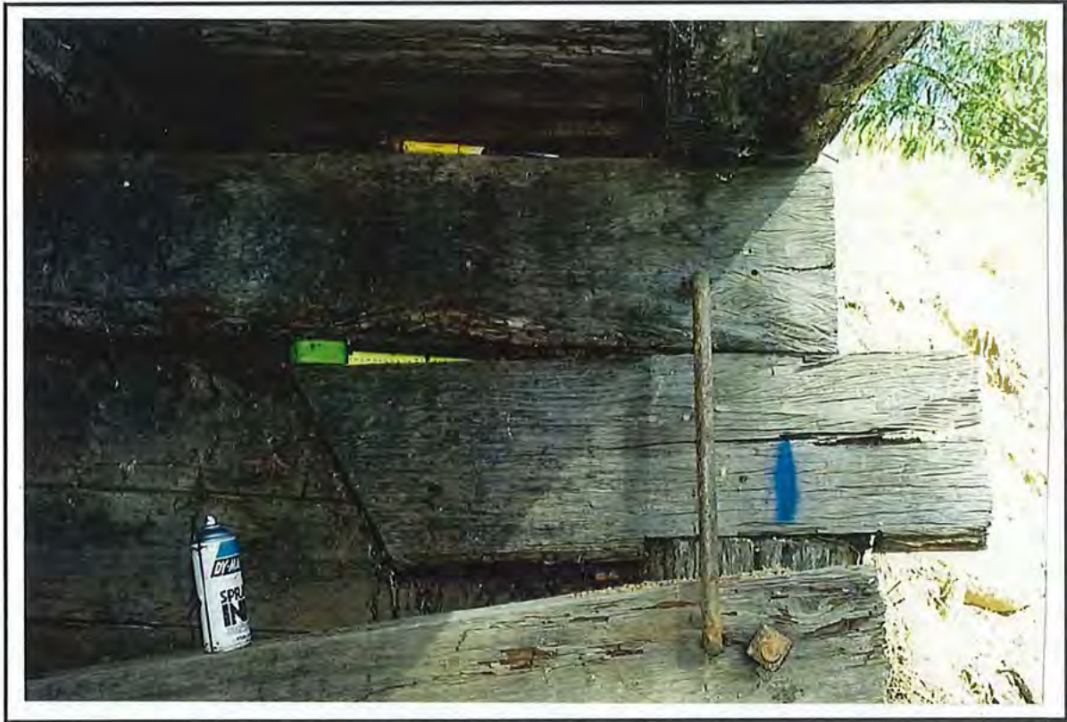
ABUTMENT 1 CORBEL 1 TILTED
