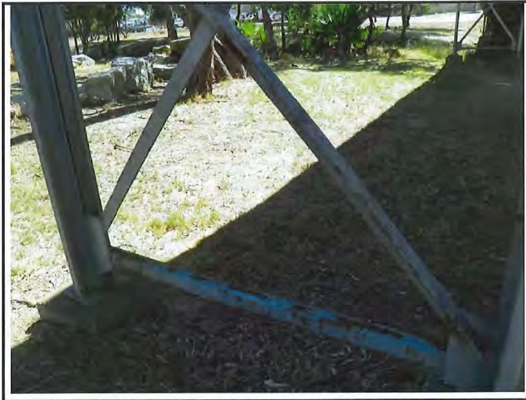
Photo No. 37: Typical surface corrosion to Piers
