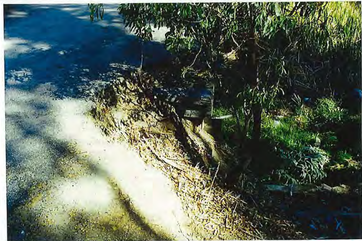
MAJOR SCOUR AT ABUTMENT 2 LEFT HAND SIDE APPROACH-FROM ABUTMENT 2 END
