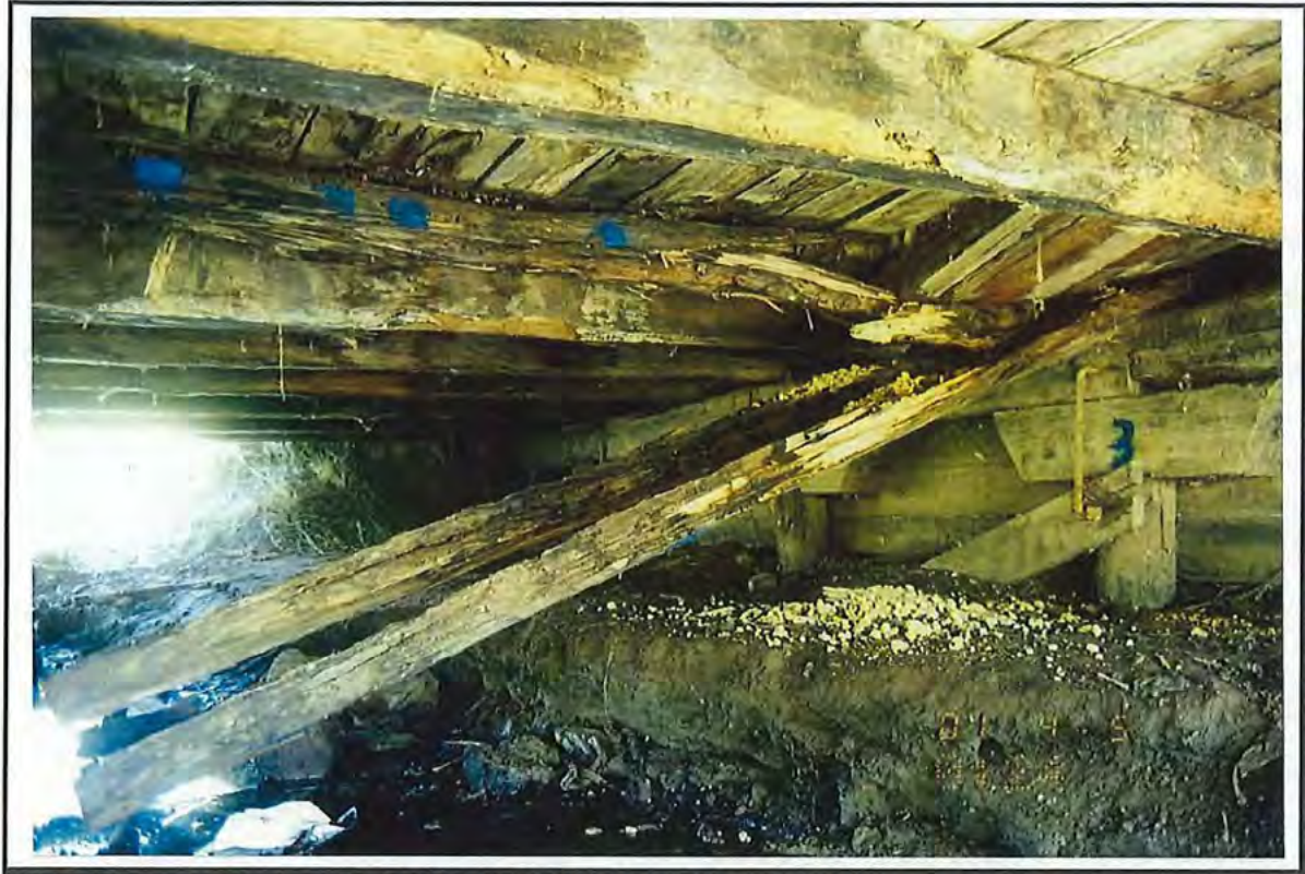
STRINGER 5 SPAN 1 SPLIT &amp; BROKEN
