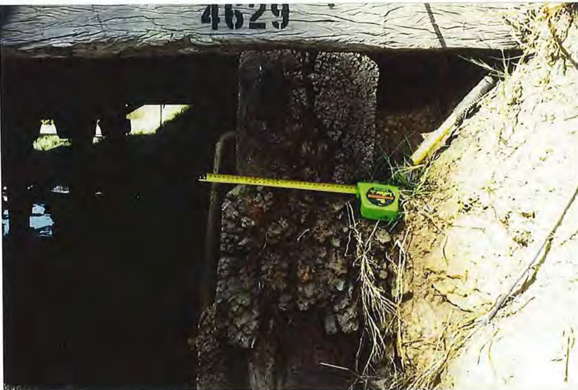
ABUTMENT 1 CORBEL 1 LEFT HAND SIDE END CONDITION - NB FULL CAP
