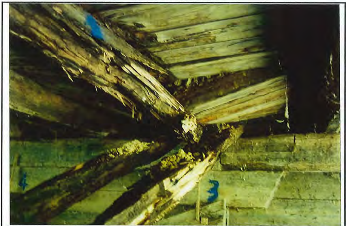
DECKING COLLAPSED AT STRINGER 5 ABUTMENT 1 END
