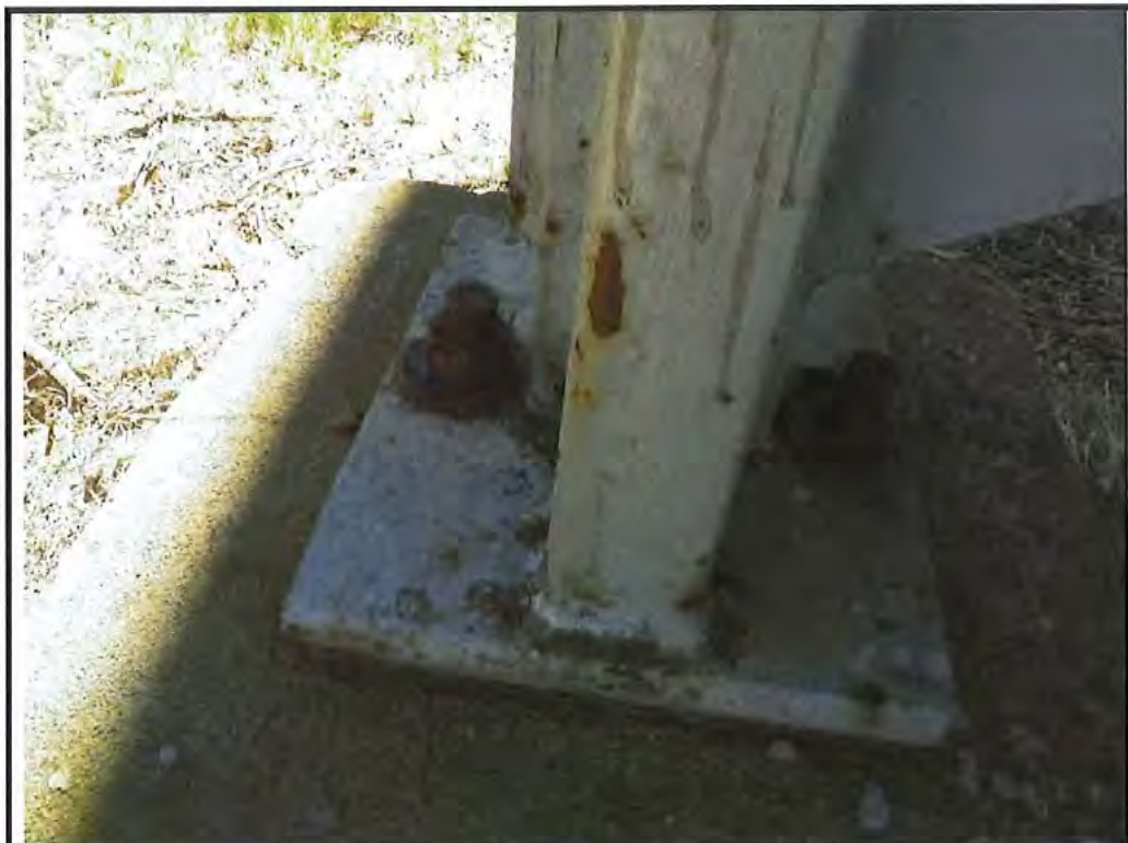
Photo No. 36: Bolts Pier 7 badly corroded – sheared off
