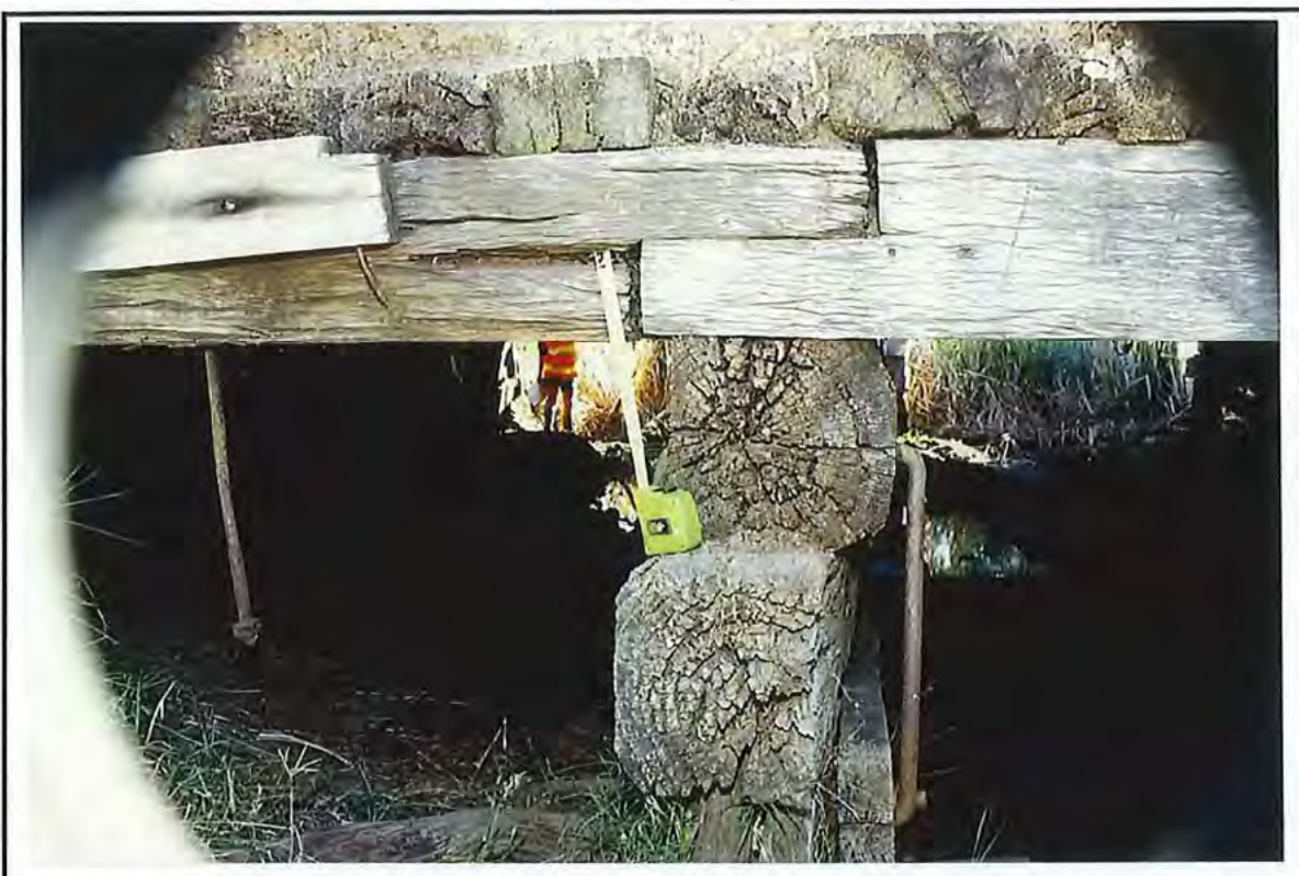
PIER 1 RIGHT HAND SIDE END CONDITION - NB STRINGER 11 END LARGE HORIZONTAL SPLIT AT CHECK OUT
