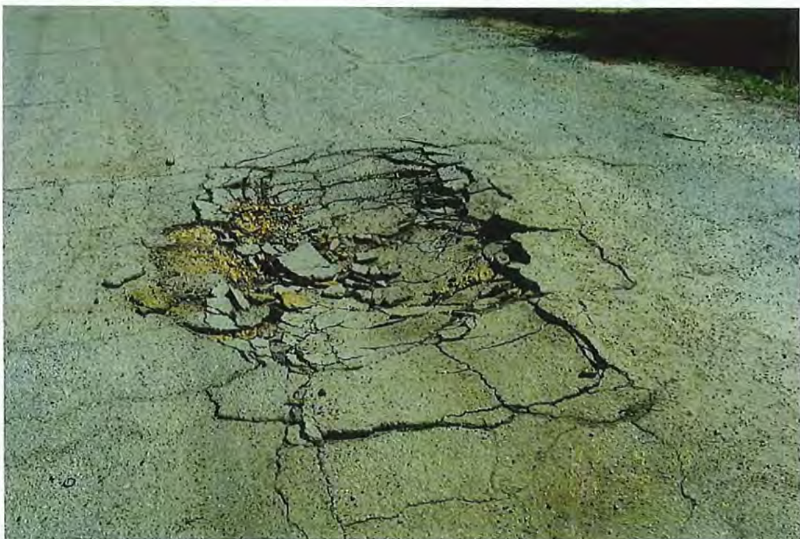
MAJOR FAILURE IN ROAD SURFACE OVER STRINGER 5 ABUTMENT 1 END Page 17
