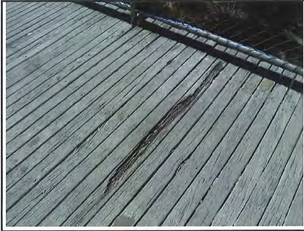
Photo No. 49: Rotten timber to deck – Span 2
