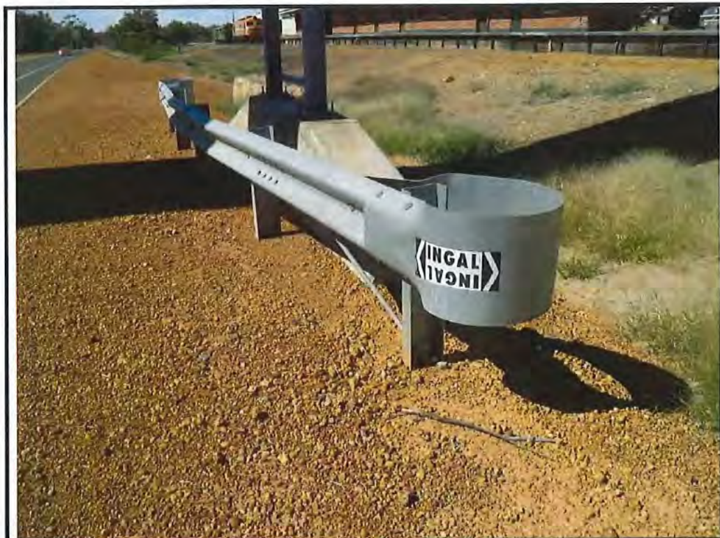
Photo No. 28: Inadequate pier protection – Pier 2
