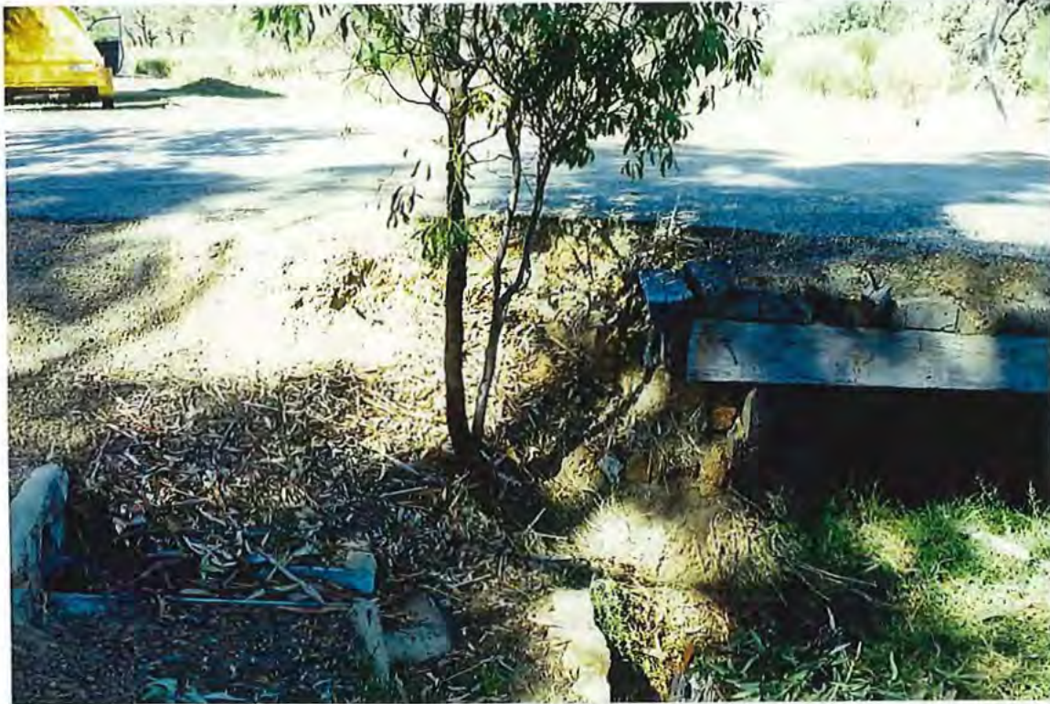
MAJOR SCOUR AT ABUTMENT 2 LEFT HAND SIDE APPROACH – FROM LEFT HAND SIDE
