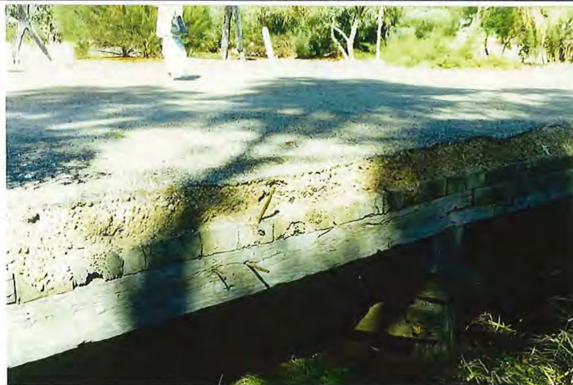
MAJOR SCOUR AT ABUTMENT 2 LEFT HAND SIDE APPROACH – FROM LEFT HAND SIDE
