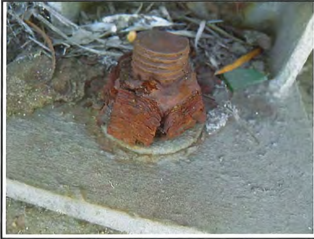
Photo No. 55: Corroded bolts to Pilaster 2
