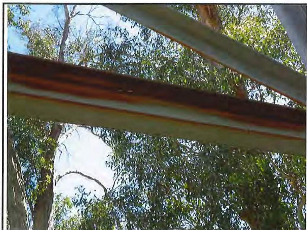
Photo No. 54: Surface corrosion to Pier 5 and 6 bracing
