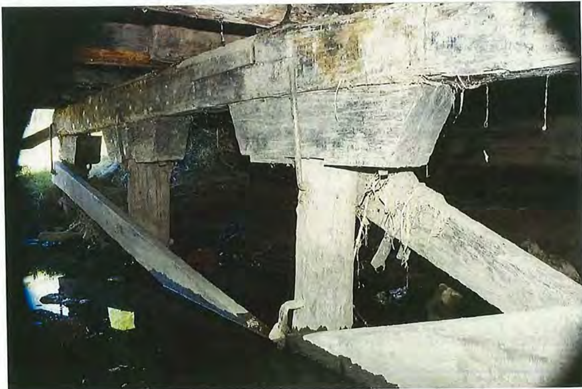
PIER 1 AT PILE 4 TIEING BARS – TYPICAL
