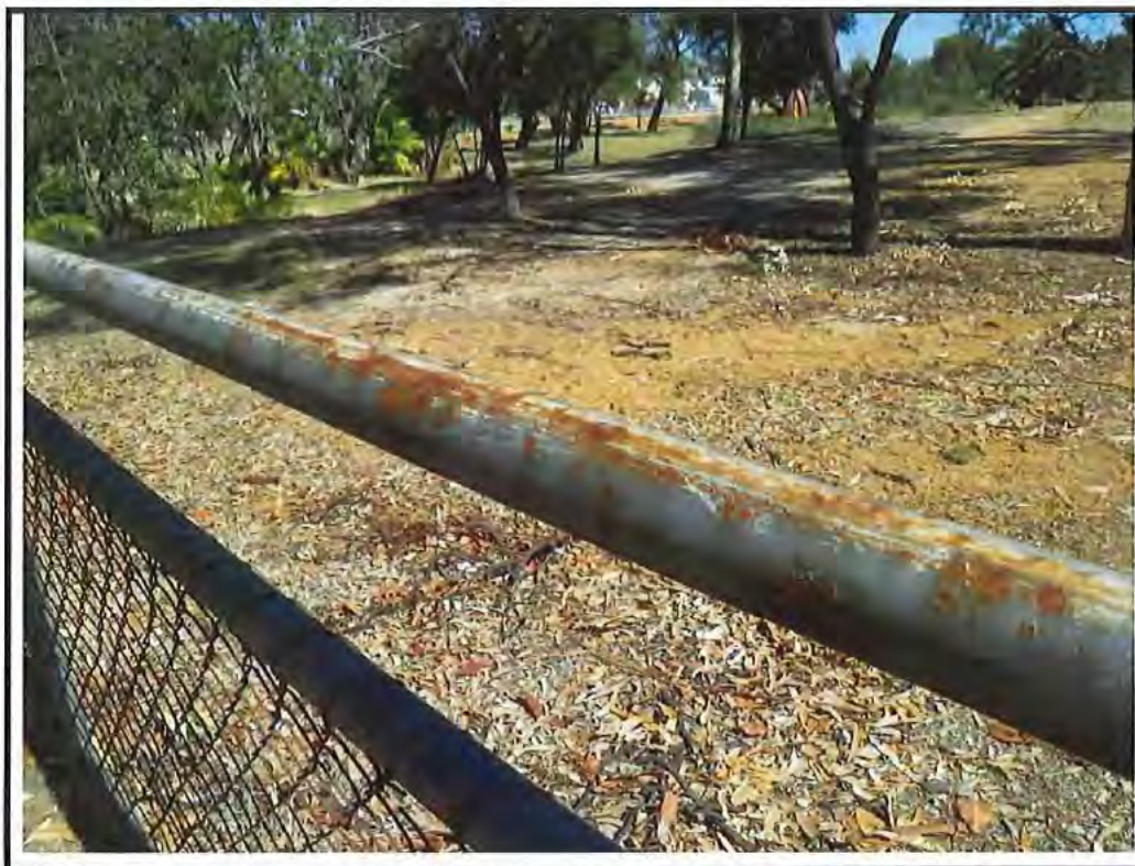
Photo No. 45: Rusting to approach 2 rails
