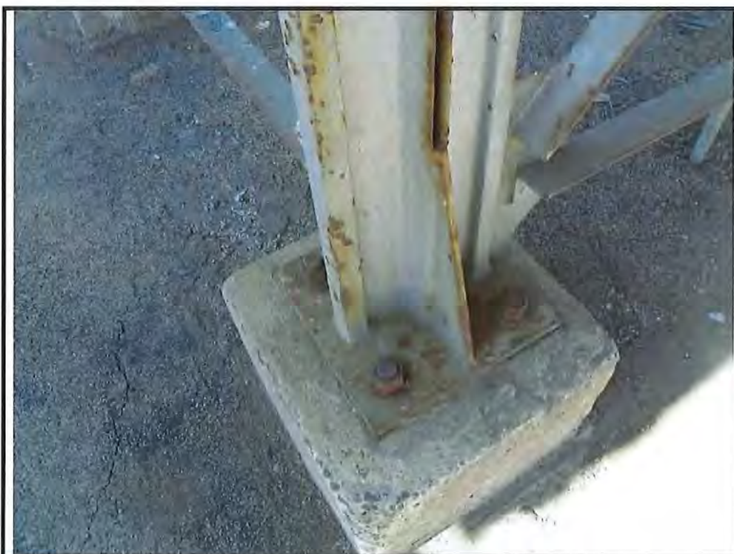
Photo No. 26: Rusting to all Pilaster 1 bolts – minor surfacing rust to steel
