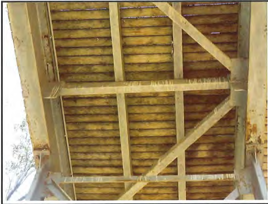
Photo No. 33: Minor surface corrosion common throughout
