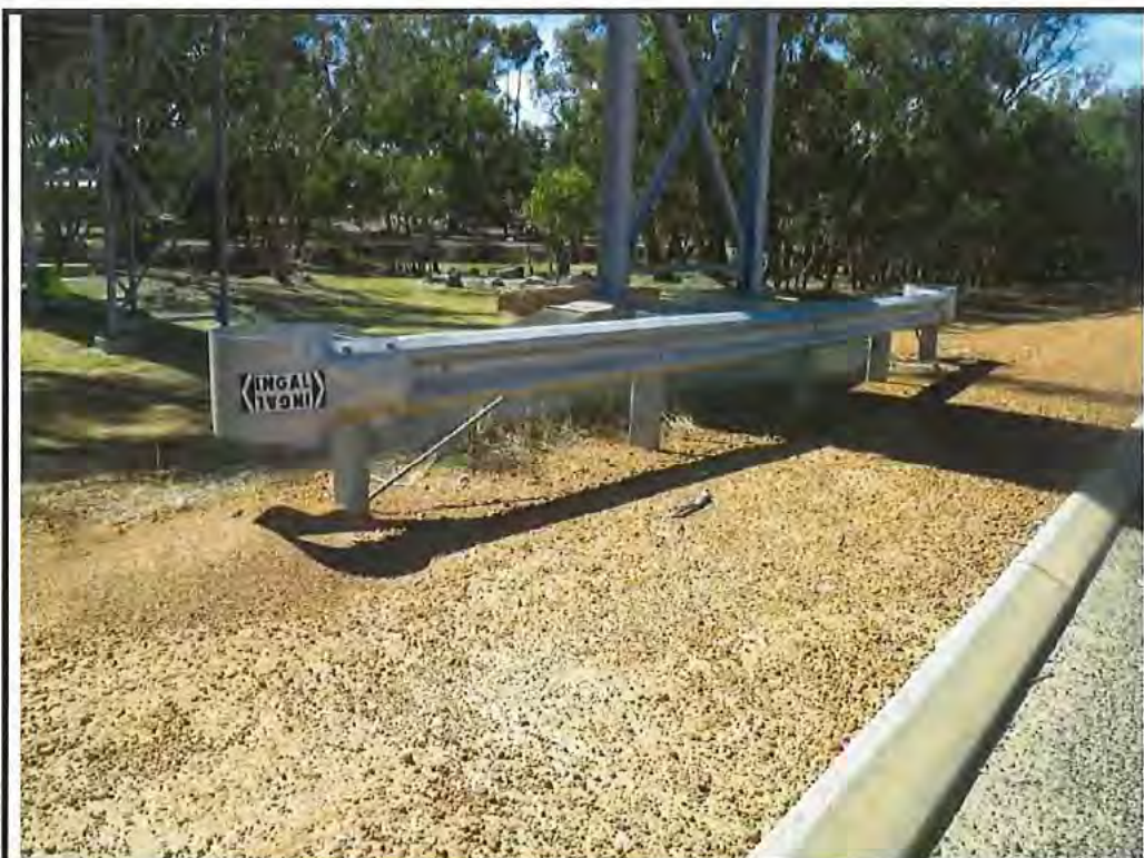
Photo No. 30: Inadequate pier protection – Pier 4
