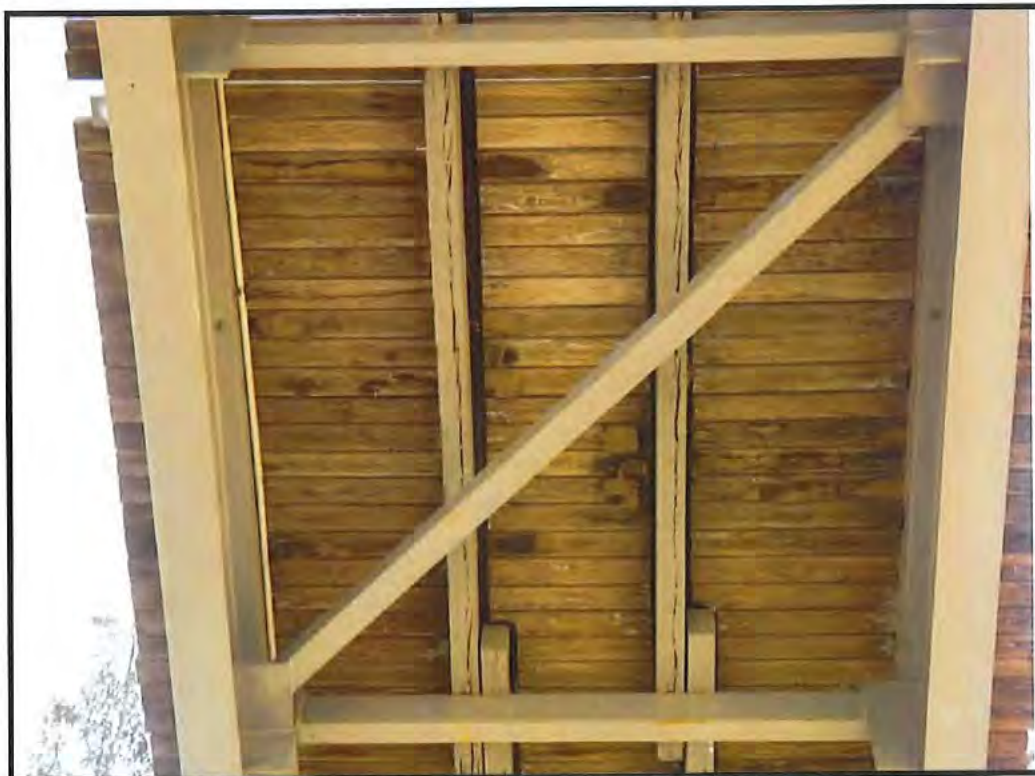
Photo No. 32: Timber bearing split
