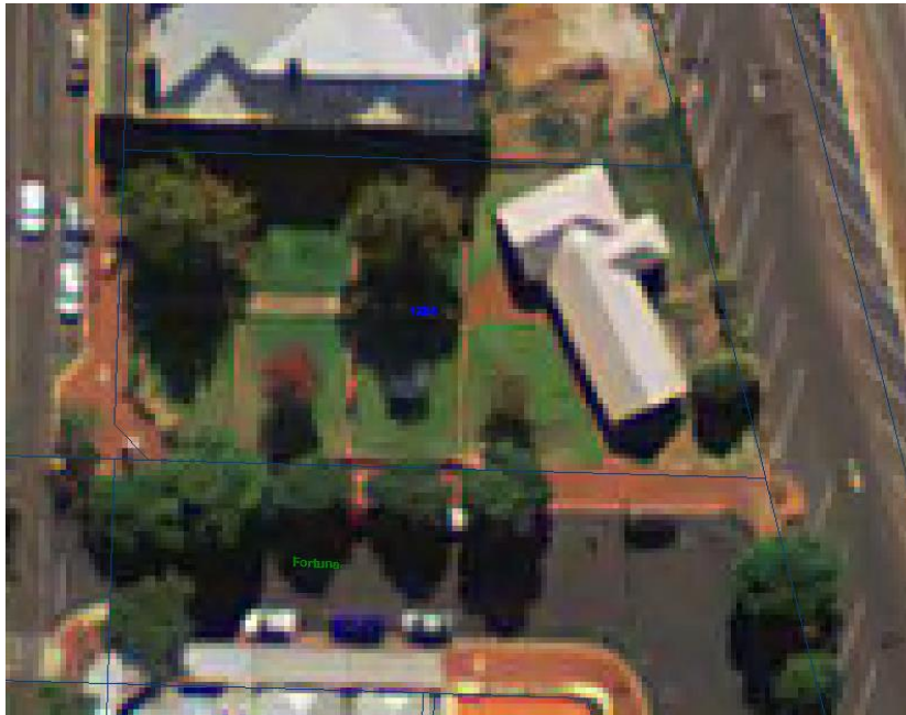
Figure 1 Mackie Park Reserve showing the offices and ablutions
