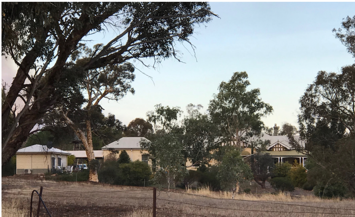
Rosedale Road frontage
