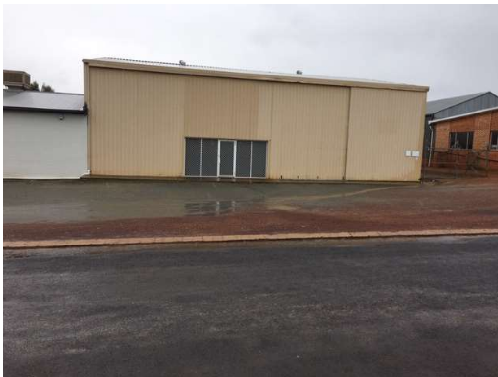
Photo 3: Generous on-site parking
