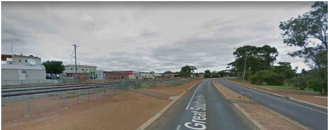
Figure 4 View of pedestrian access on northern approach
