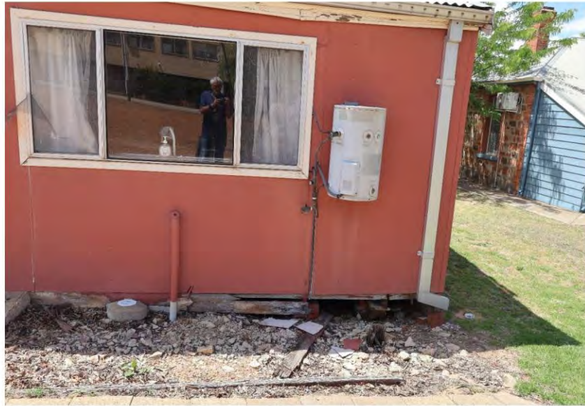
FIGURE 5A & B: SURFACE WATER SHOULD BE PREVENTED FROM ENTERING IN UNDER THE BUILDING.
