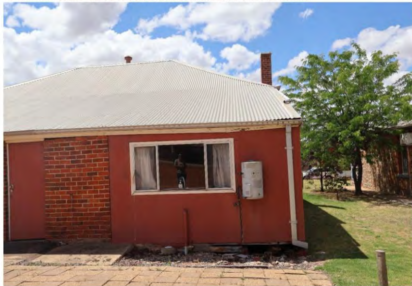
FIGURE 5A & B: SURFACE WATER SHOULD BE PREVENTED FROM ENTERING IN UNDER THE BUILDING.
