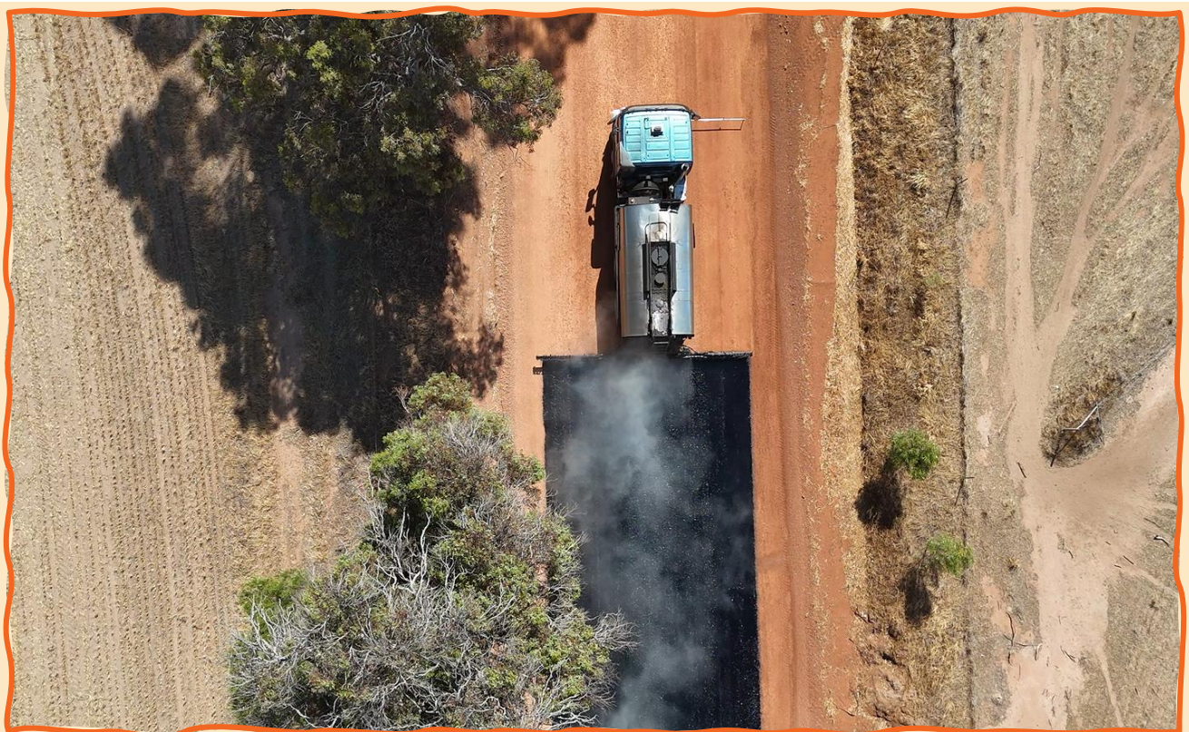
WHINBINROCK ROAD SEAL PROJECT
