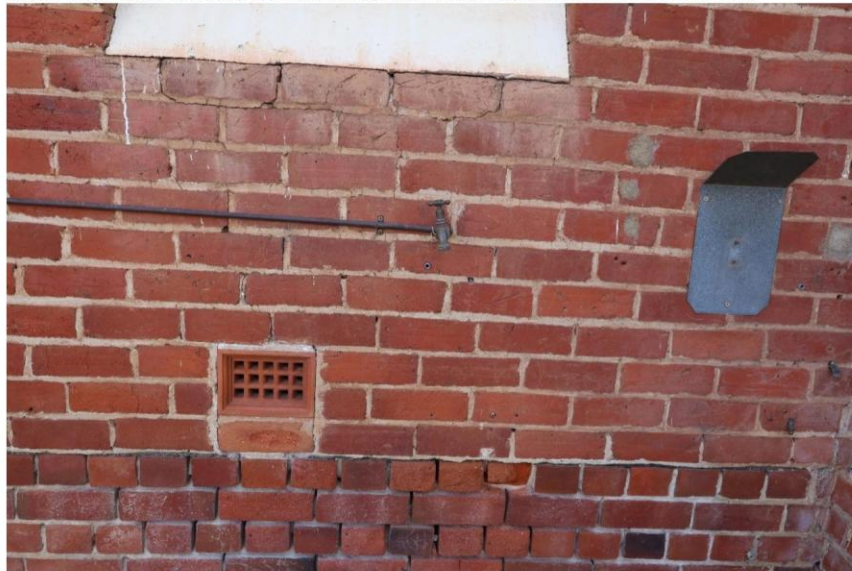
FIGURES 4A & B: BRICKWORK COULD BE RE-POINTED. SURFACE WATER SHOULD BE DRAINED AWAY FROM THE WALLS.
