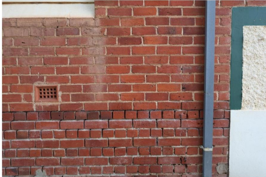
FIGURES 4A & B: BRICKWORK COULD BE RE-POINTED. SURFACE WATER SHOULD BE DRAINED AWAY FROM THE WALLS.
