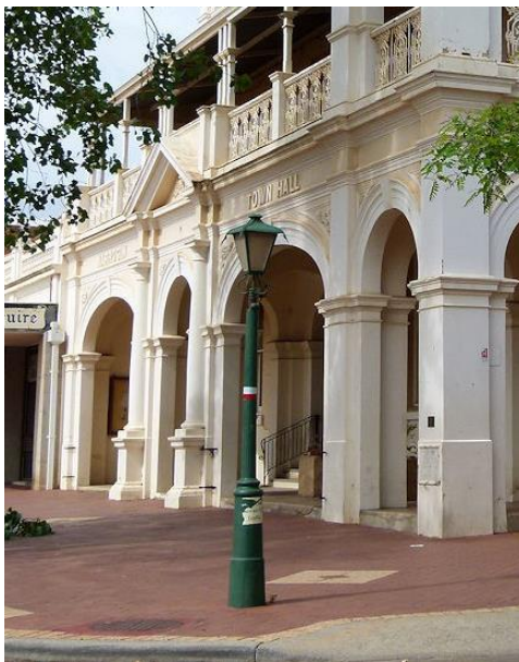
Figure 2 Image of existing pole suggested for replacement.
