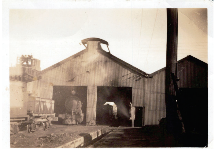
From Days Gone By – The Locomotive Sheds at Narrogin Railway Station. 1948 - 1950
