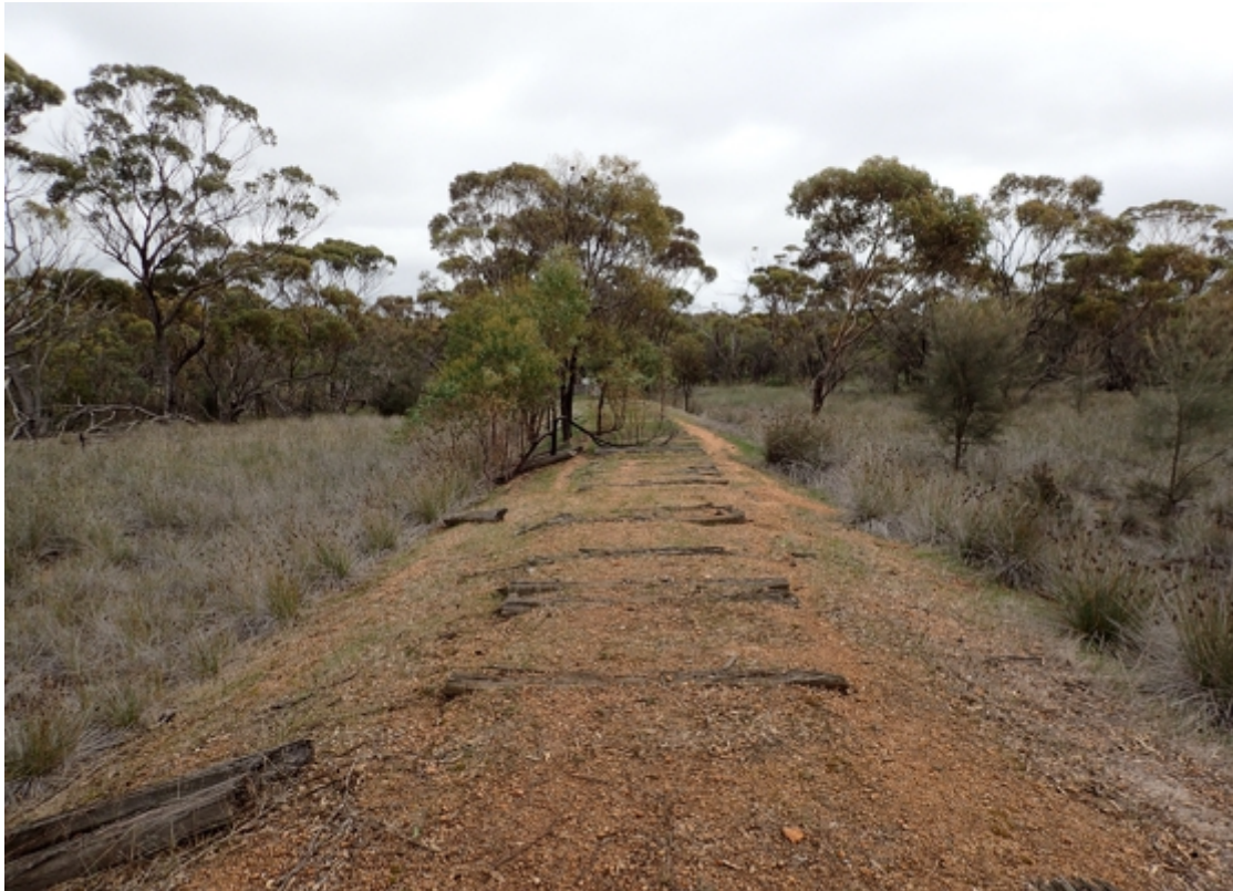
Most, but not all, of the old railway sleepers have been removed from the disused railway.
