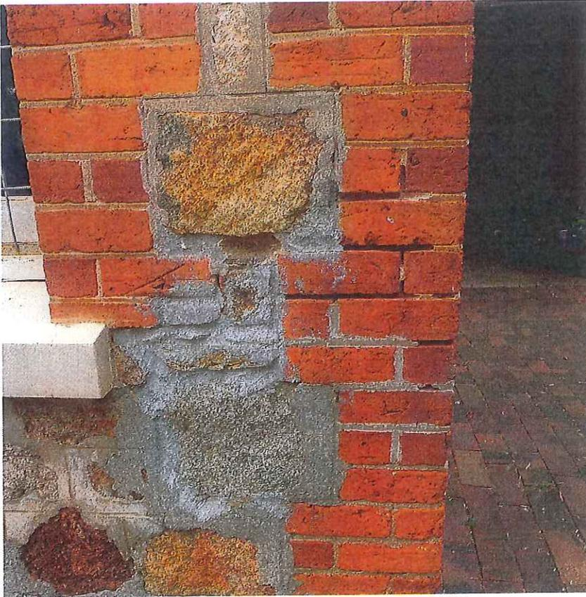
Detail of north corner of east wall showing cement interventions and fretted mortar on the face bricks.
