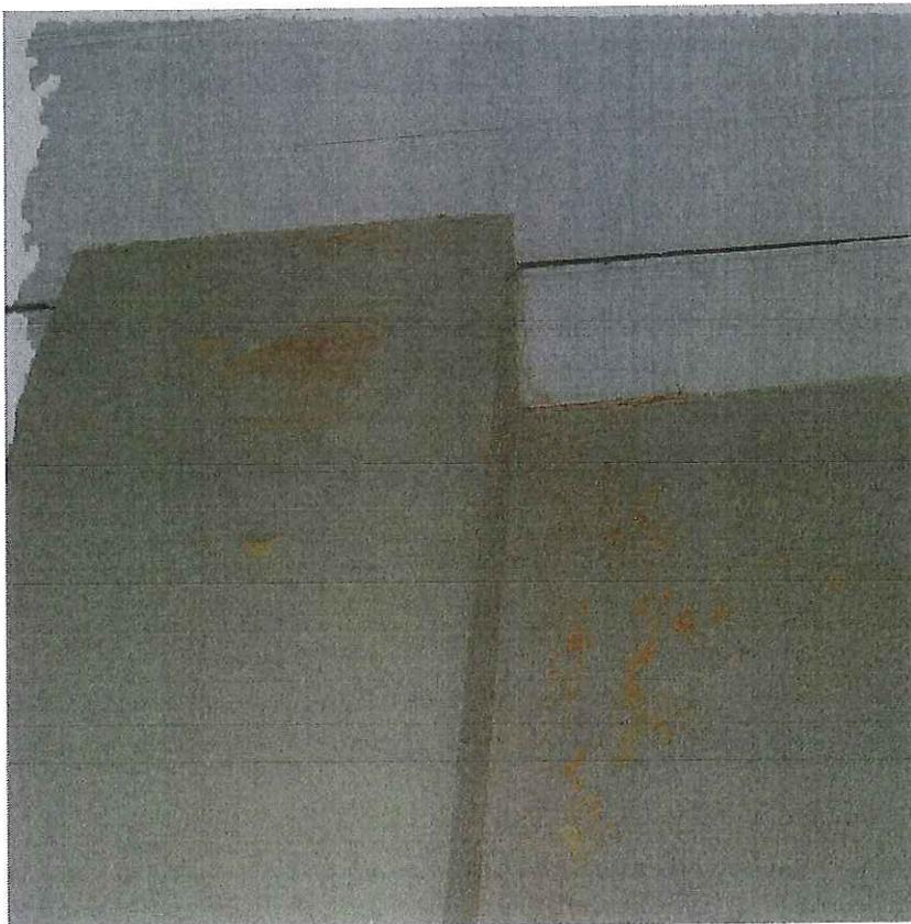
Interior: The chimney on the east wall of the 1894 school room, showing evidence of falling damp.
