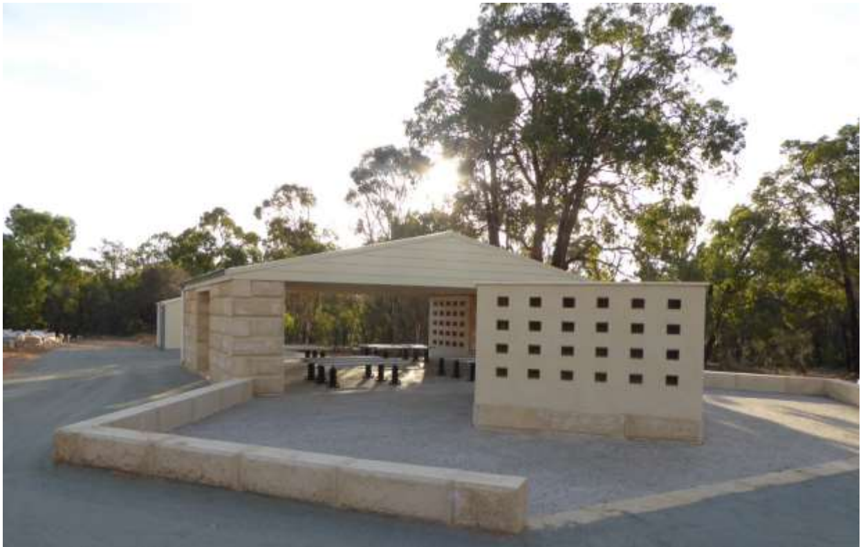
During the period, the first phase of the niche wall at the Narrogin Cemetery was completed.
