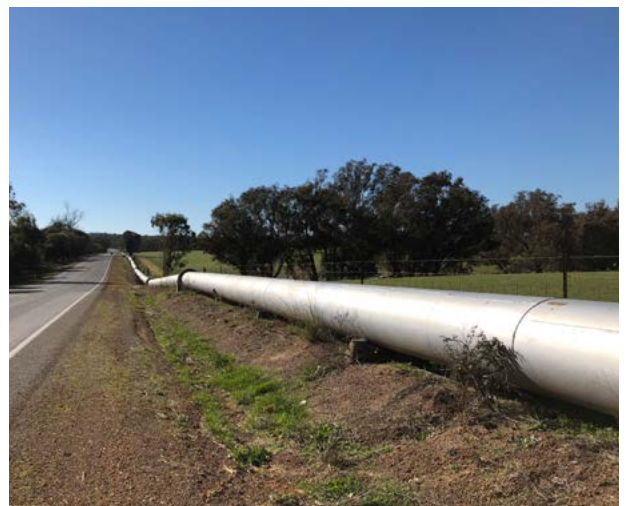
The Williams to Narrogin water pipeline | Photo Penny Bovell
