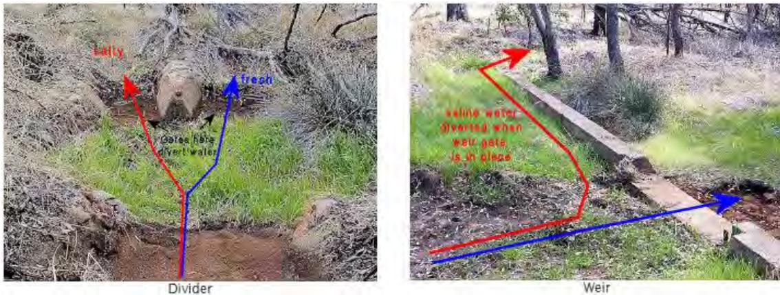
Plate 3: The historical drainage network installed at Railway Dam Reserve (Sawkins 2017)
