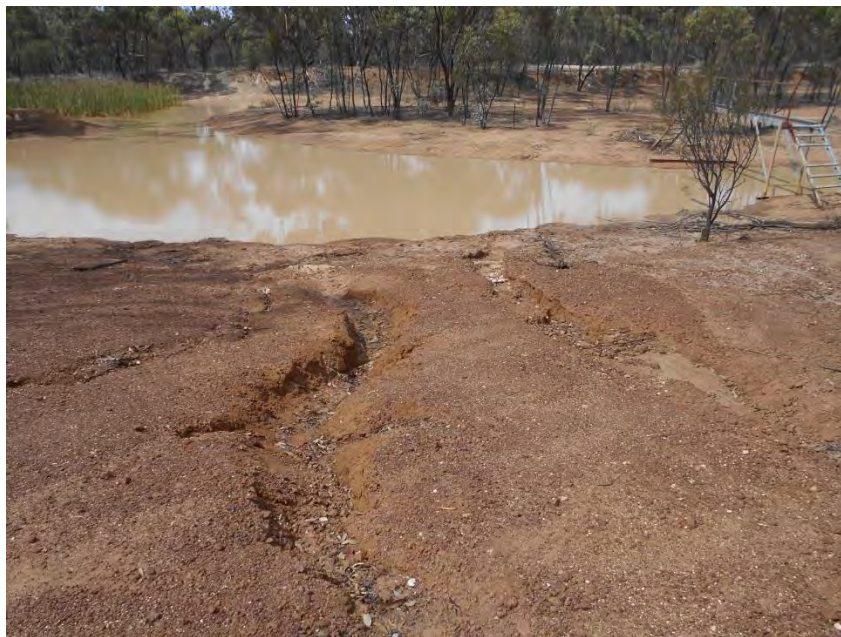
Plate 2: Erosion (and bridge) at Archibald Park
