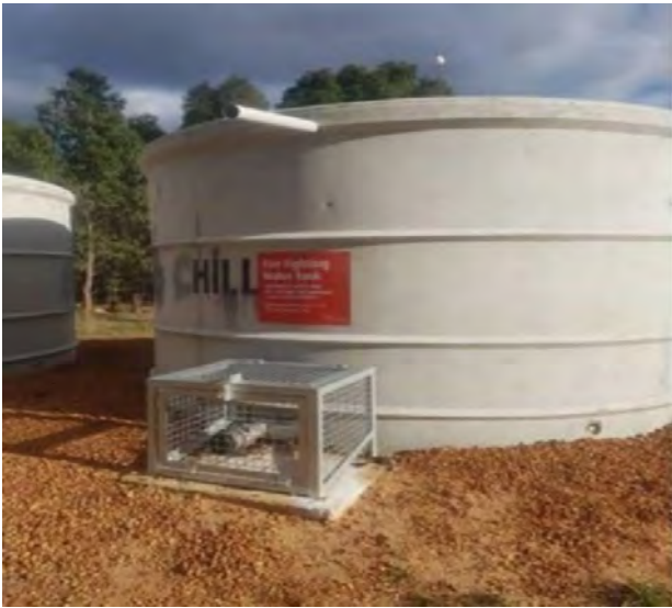
Strategic 47,000 Litre Concrete Tank & Protected Fittings
