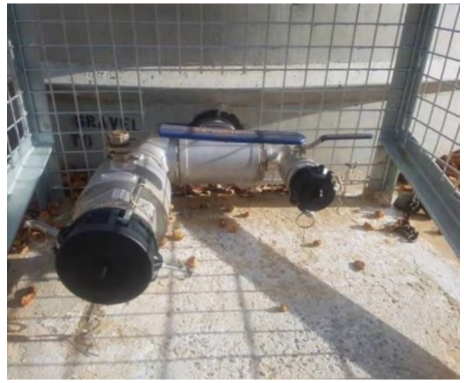
Strategic 47,000 Litre Concrete Tank & Protected Fittings
