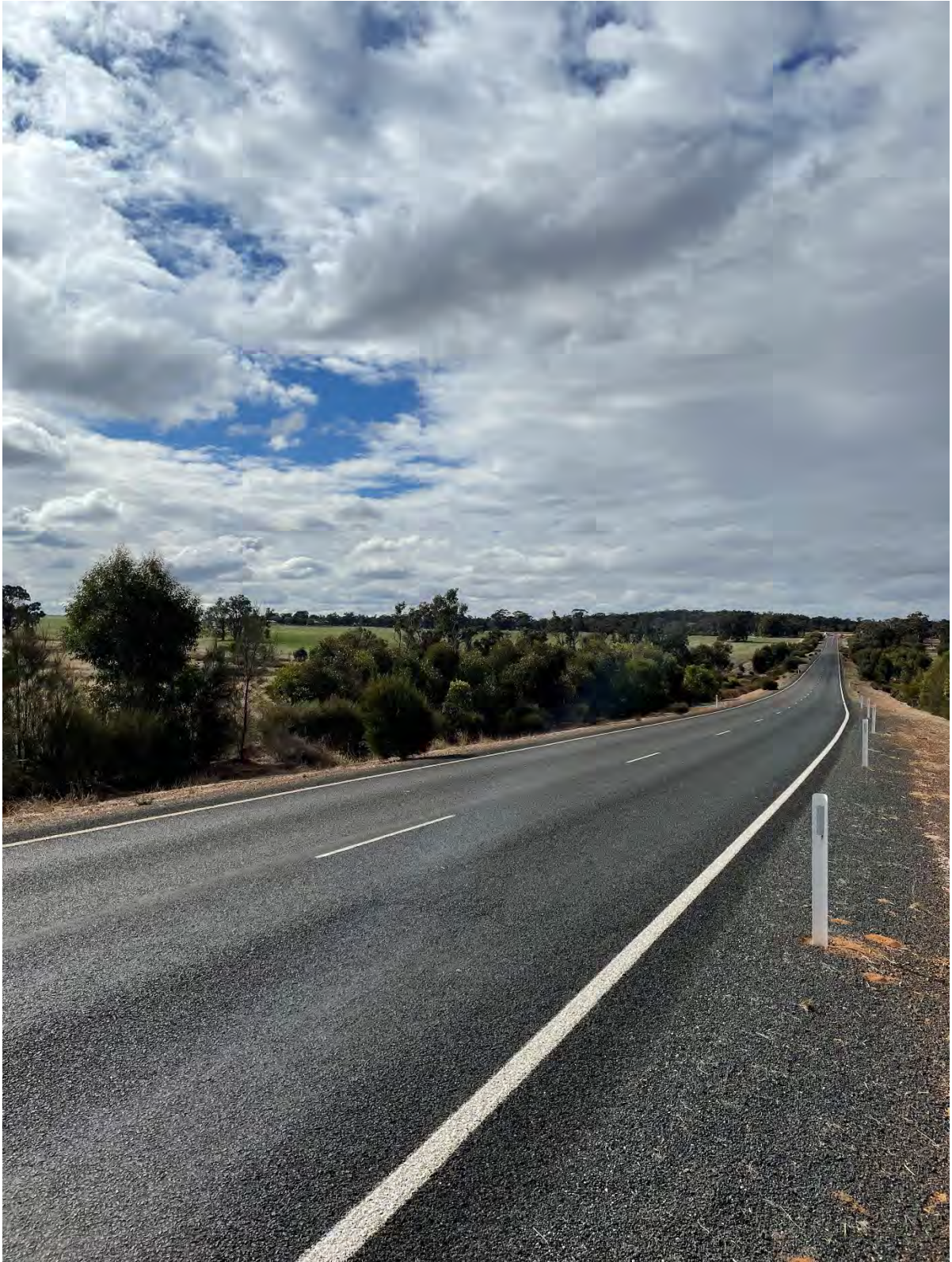
Figure 6 - Lot 31 Great Southern Highway viewed from Wanerie Road facing east, approximately 500m west of the biorefinery site (source: Rise Urban 2022)
