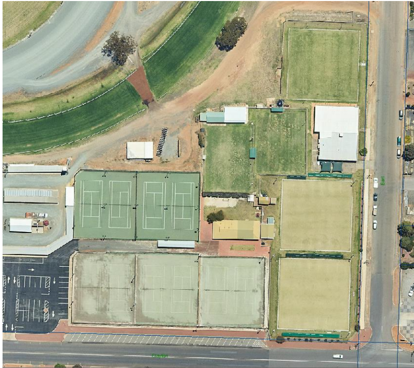
Figure 1 12 Tennis Courts to the east of the NRLC Building
