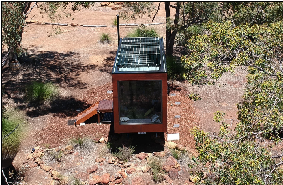
Roof-Mounted Solar Panels
