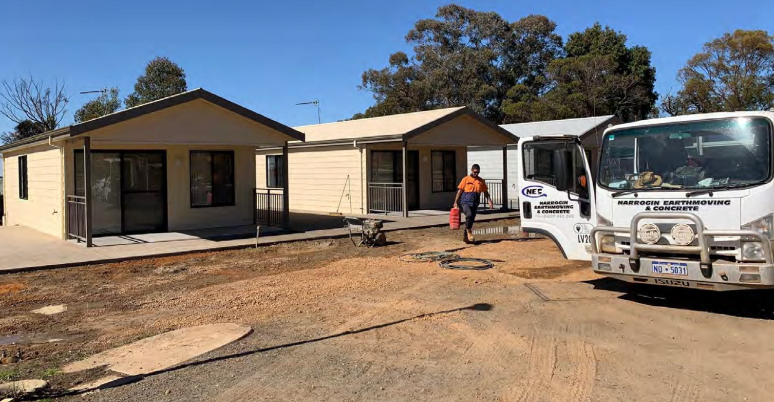
The construction of three Accessible accommodation units at the Narrogin Caravan Park
