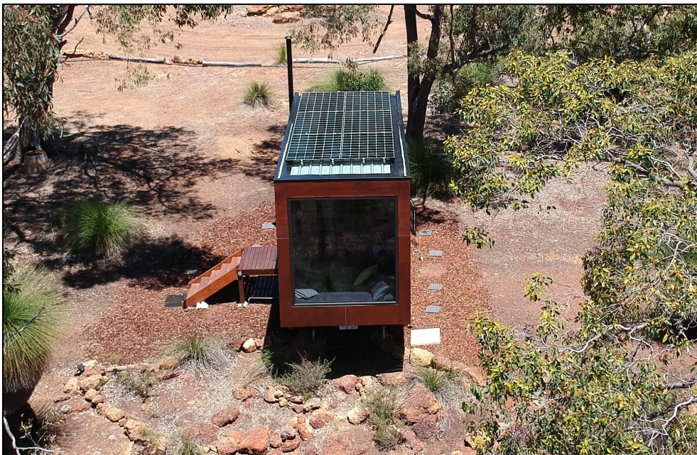
Roof-Mounted Solar Panels
