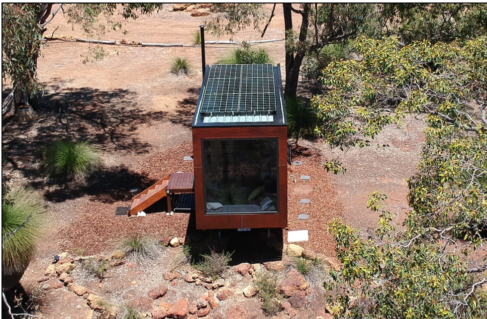
Roof-Mounted Solar Panels
