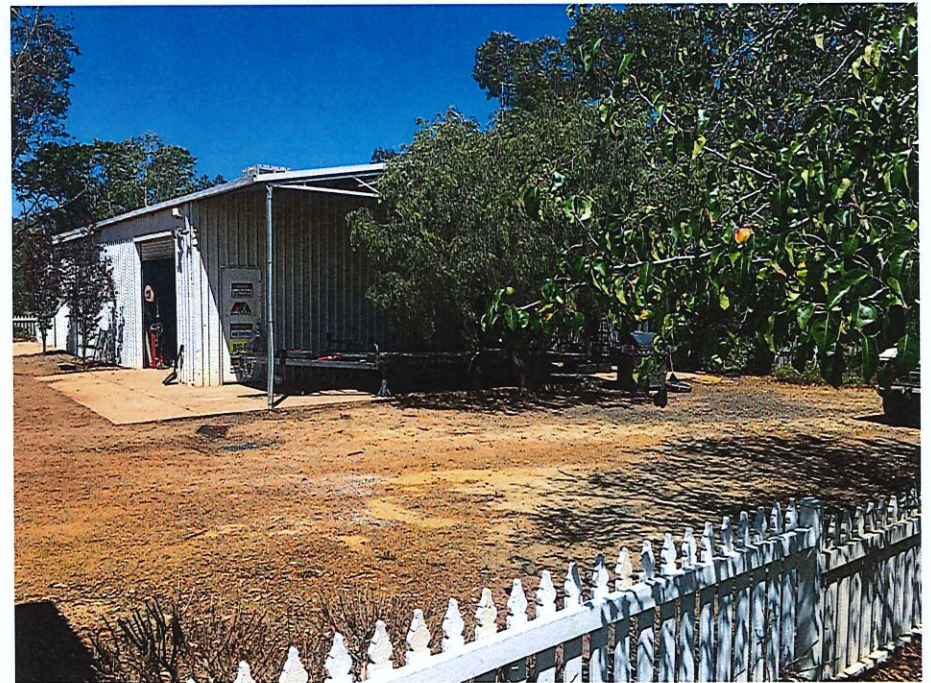
view from house - looking SW
