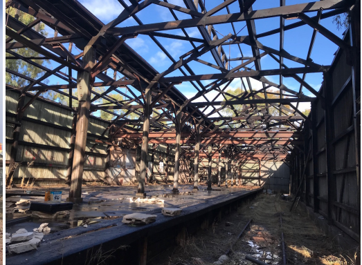
Northam goods shed – partially demolished with removal of asbestos roof.
