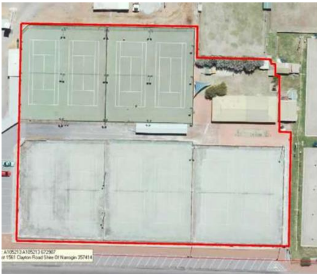
Tennis complex on Clayton Road
