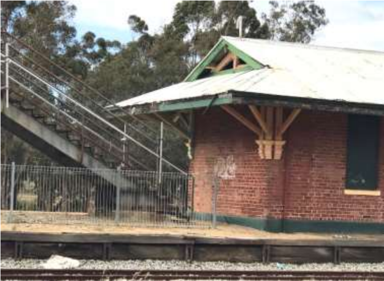
Photo 10 Narrogin Railway Station View of the north end access to the platform from the stairs off the pedestrian overpass.
