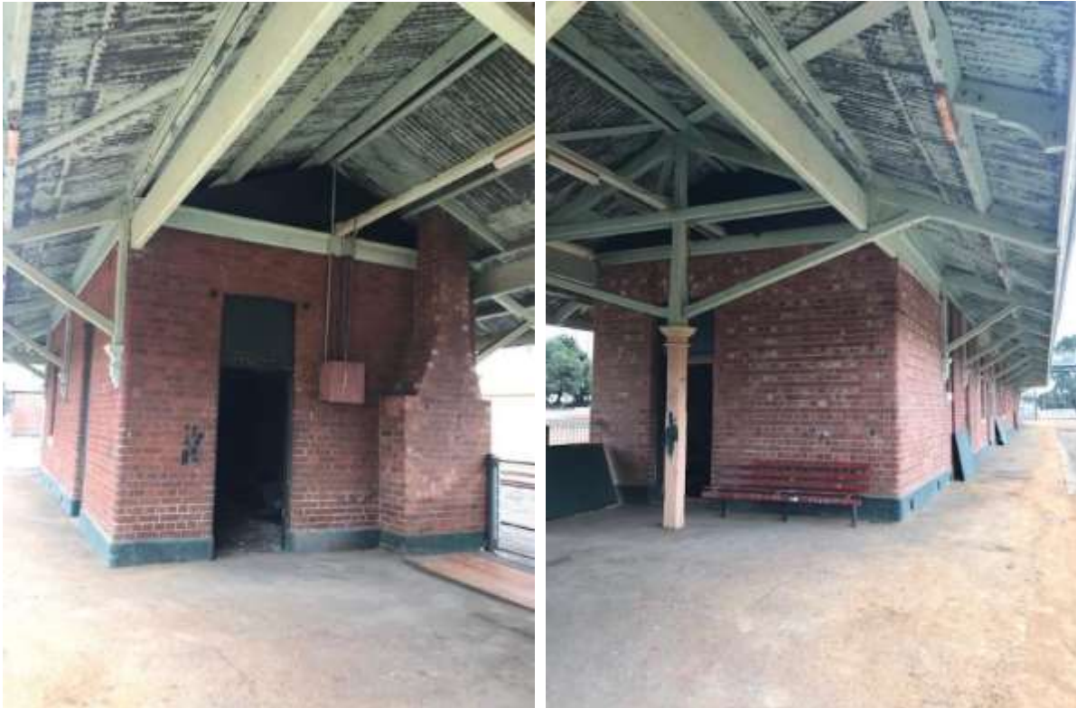
Photos 21, 22 Narrogin Railway Station The north wall of the former refreshment room (looking south) , and on the other side of the open space is the south wall of the main station building (ladies waiting room) looking north. Both looking along the east side.
