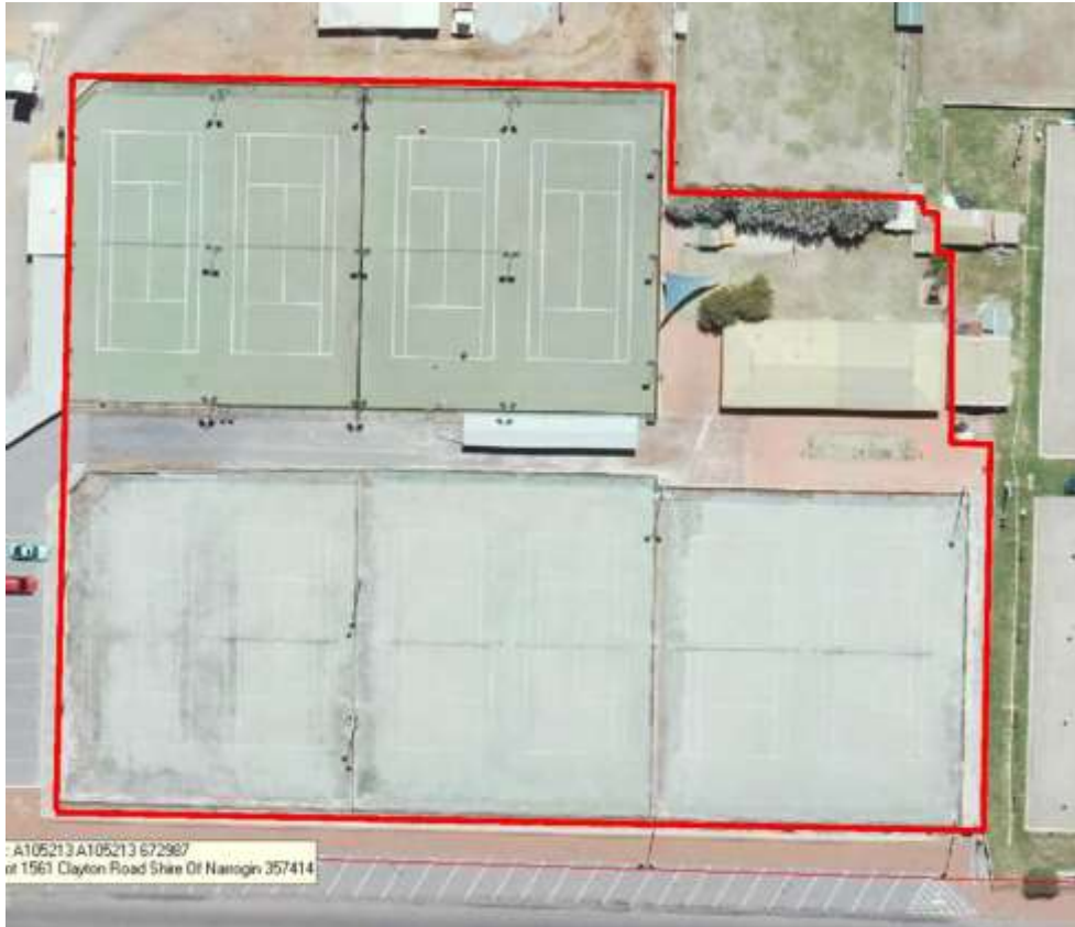
NTC courts proposed for resurfacing.
