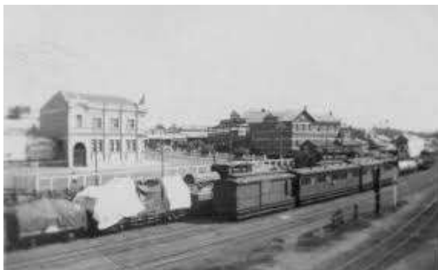
Railway yard with town and the Horden Hotel in the background. Unknown date.
