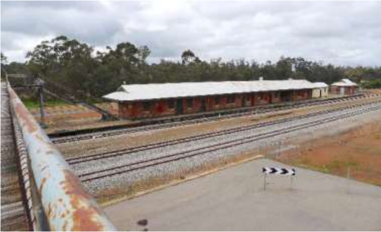
Photo 4 Narrogin Railway Station View looking southeast from the pedestrian overpass.
