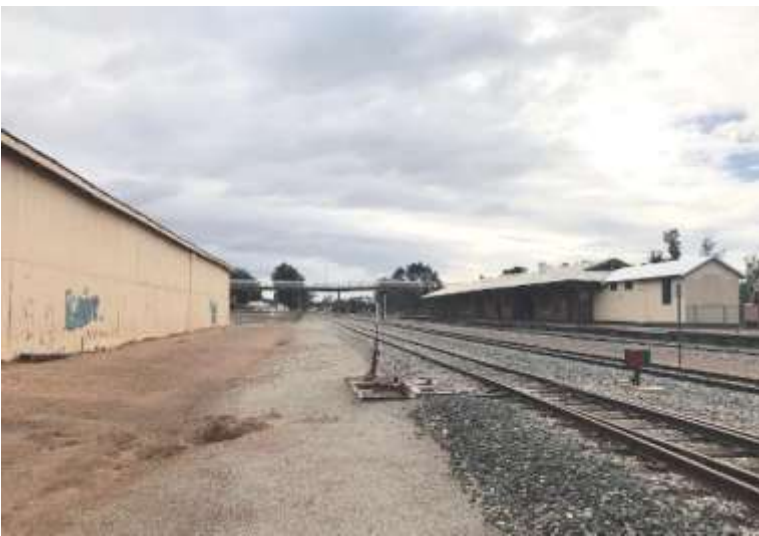
Photo 5: Narrogin Railway Station & Goods Shed View looking north.
