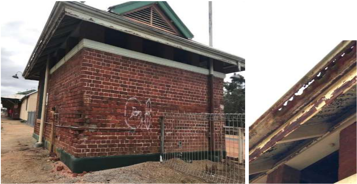
Photos 61, 62 Narrogin Railway Station Ablution building view looking northeast showing station (left) at south end of the railway station platform; and, gutter detail.
