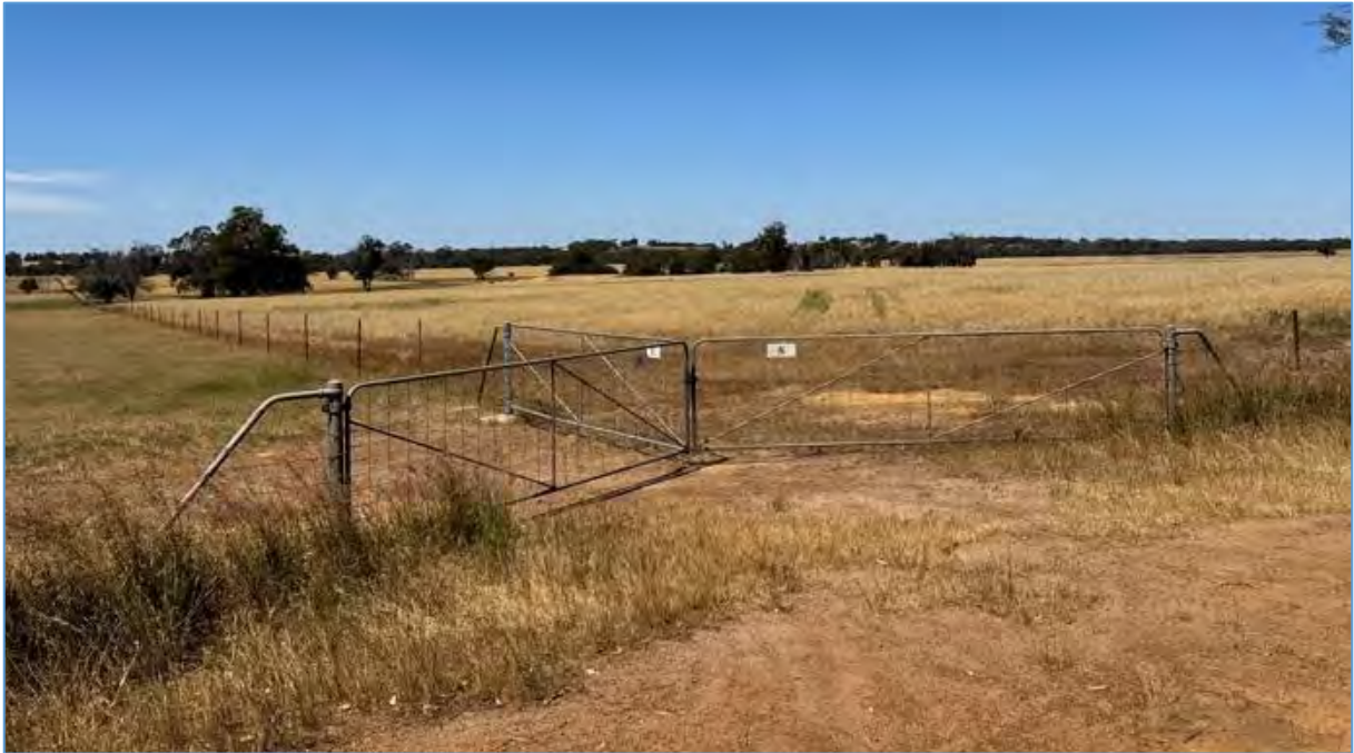
Figure 20: Southern Site Access 2 (Parks Road) – Site Photo
