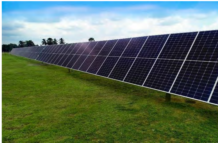
Figure 3 Single-Axis “1P” Tracking Support System
