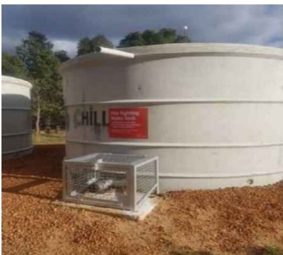
Strategic 47,000 Litre Concrete Tank & Protected Fittings
