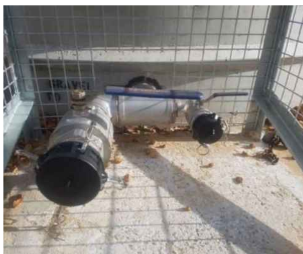
Strategic 47,000 Litre Concrete Tank & Protected Fittings
