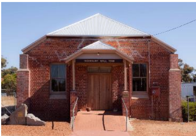
HIGHBURY DISTRICT HALL 2013
