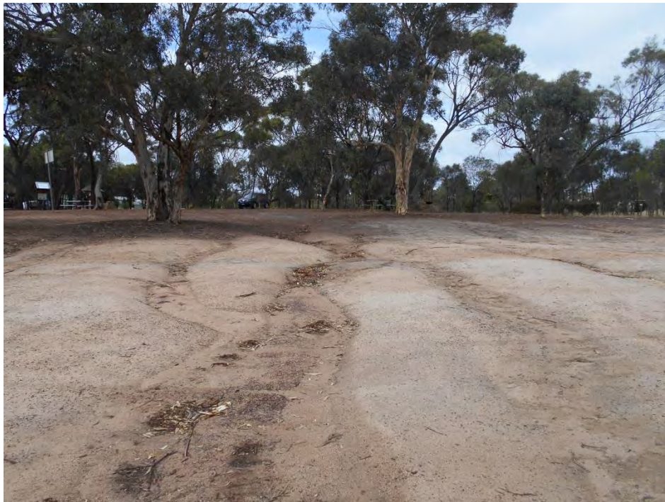
Plate 6: Erosion of banks of Railway Dam
