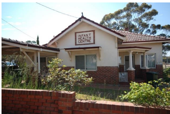
Photograph 2: The building and site are well-sited to various commercial uses including professional offices
